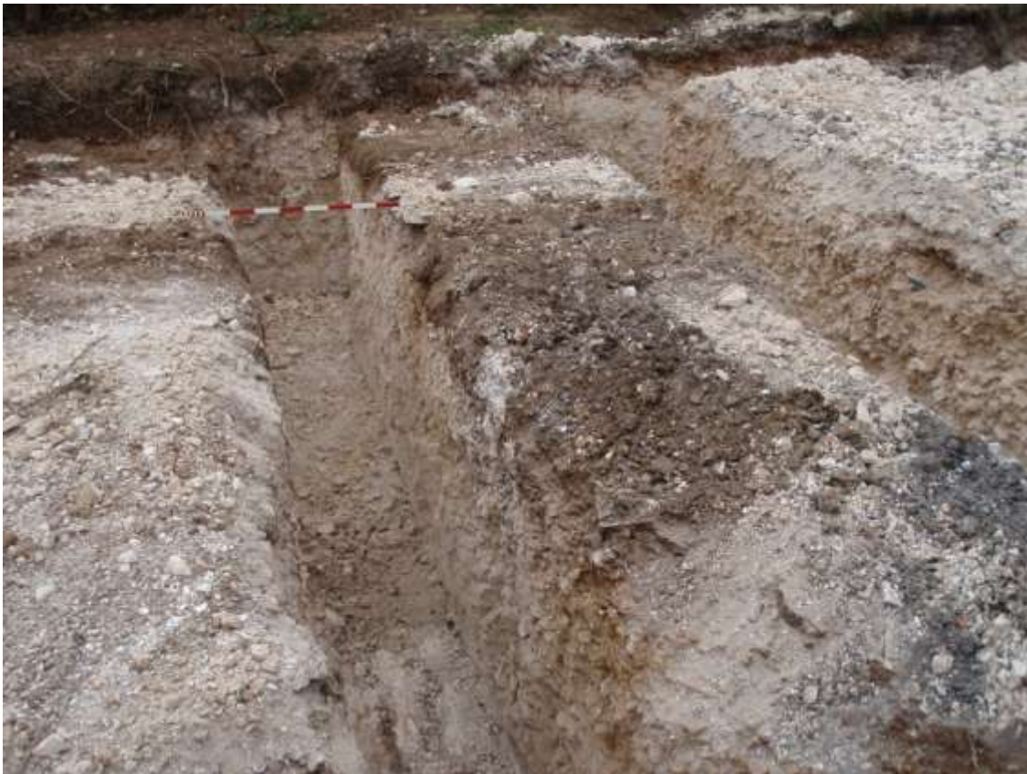
Plate 5. west foundation trenches
