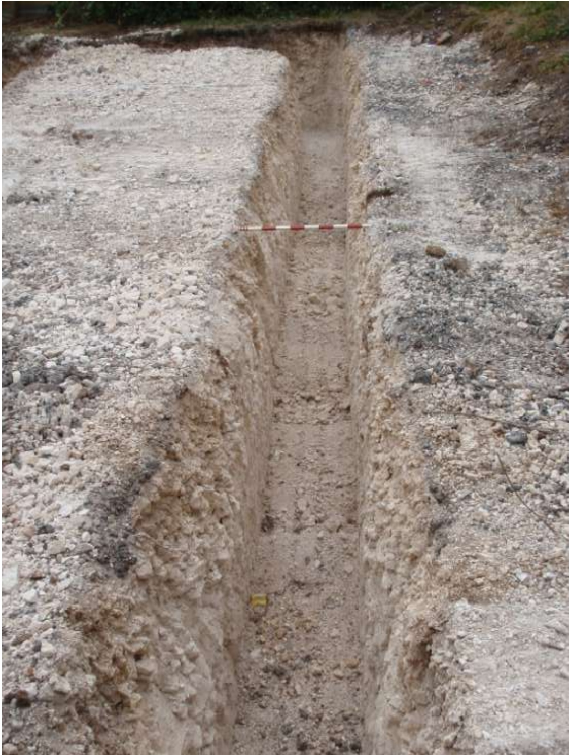
Plate 8. South foundation trenches
