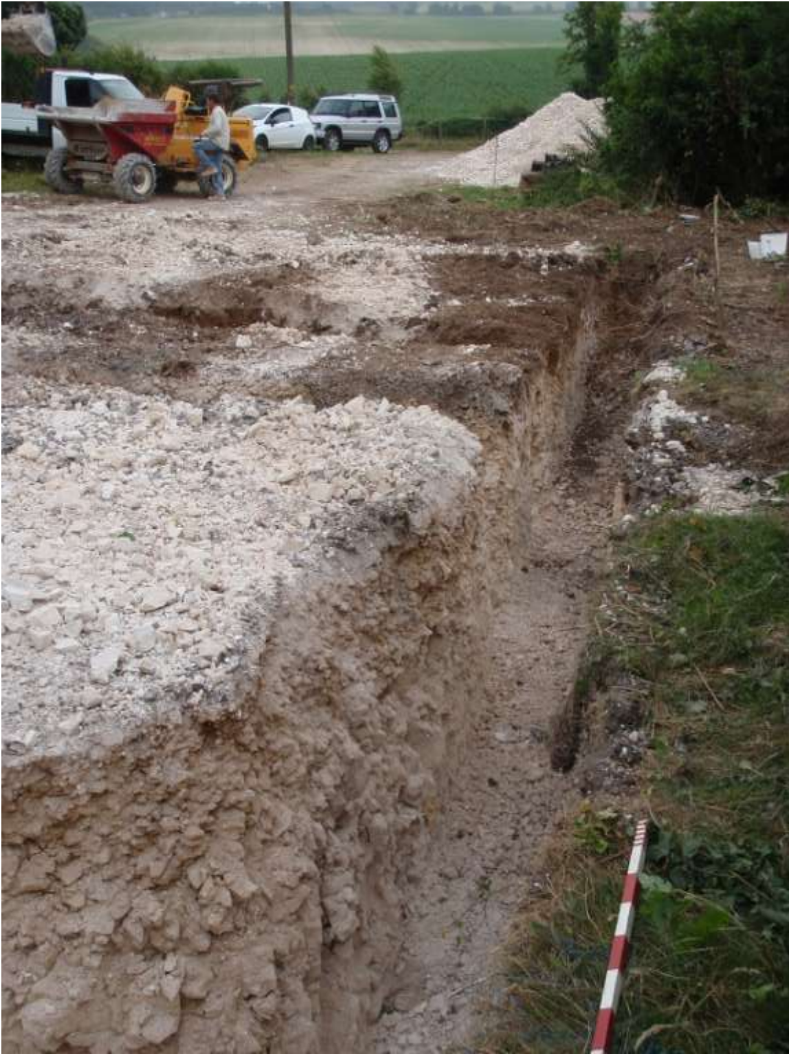
Plate 7. West foundation trenches
