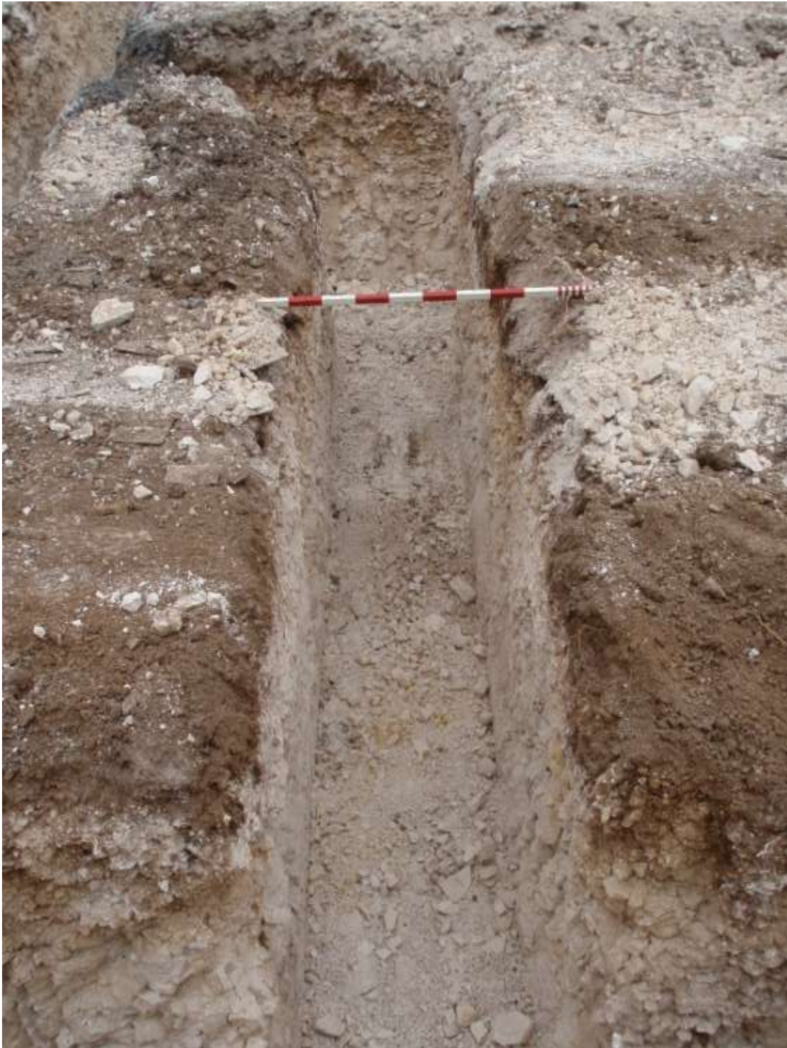
Plate 6. East foundation trenches
