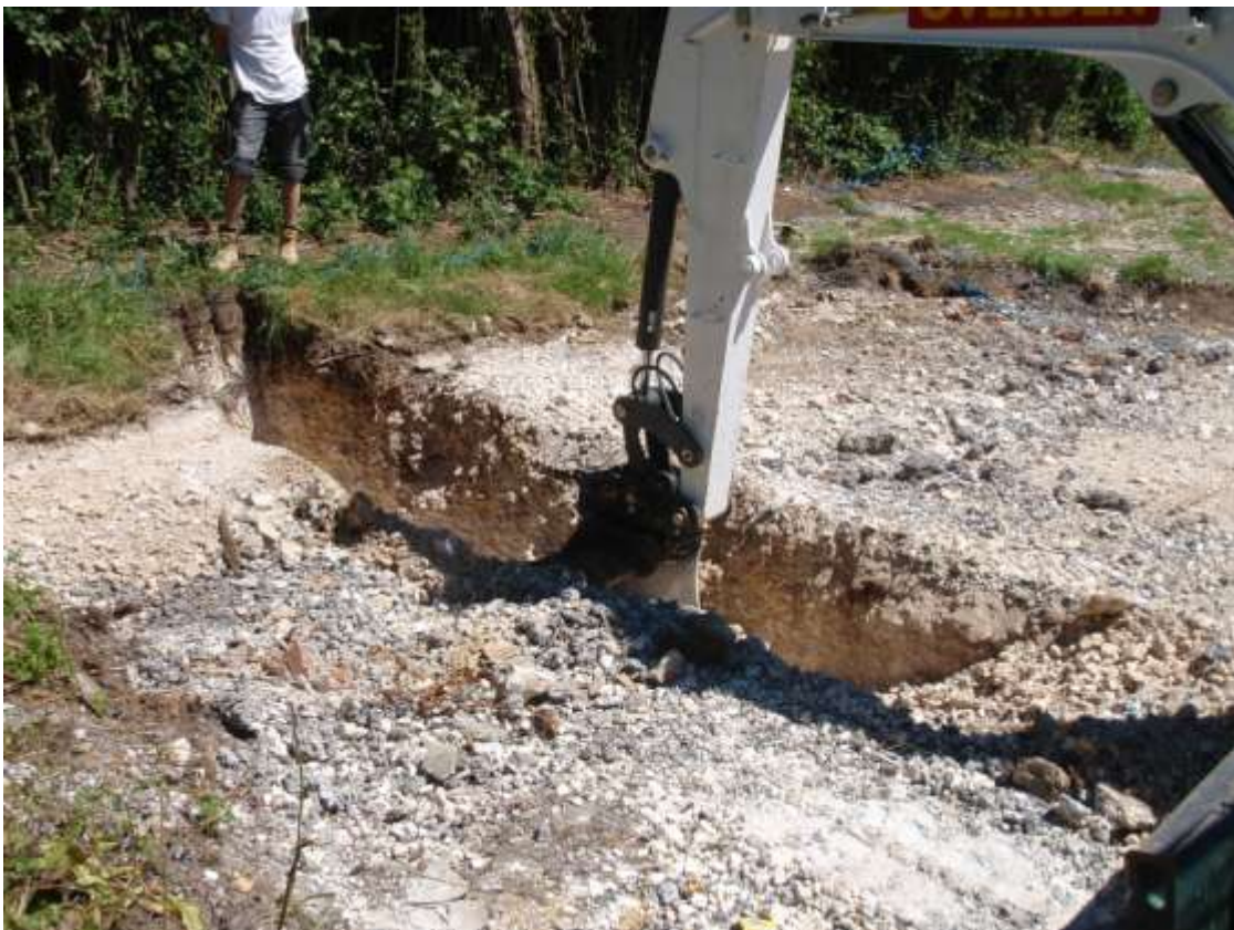
Plate 3. Cutting the first foundation trench (looking north)
